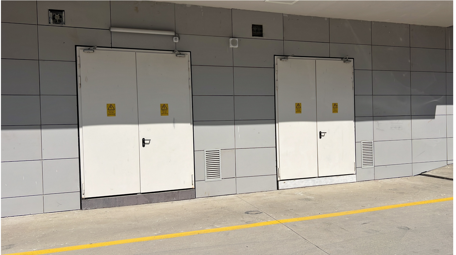
Ashgabat Pediatric Hospital, Turkmenistan, Samsun 900 bed PPP Project, Türkiye,
